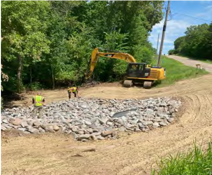
Above: Birchdale Township. This is one of five stabilization efforts the SWCD supported to prevent eroded sediment from entering Sauk Lake along Alcott Drive.
