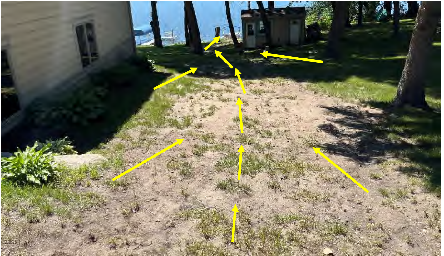
Top of slope looking down towards lake, arrows showing movement of water down to lake
